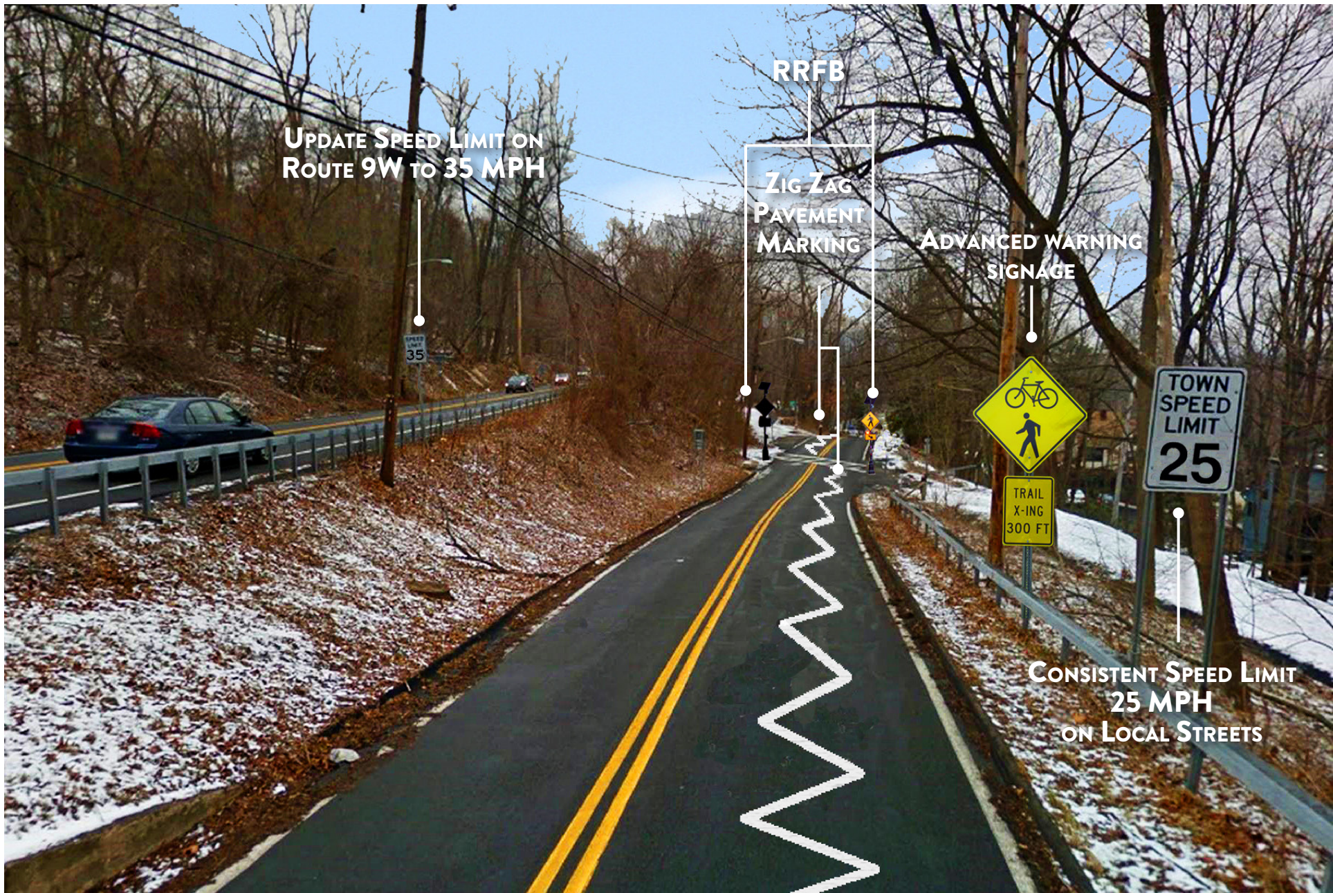
View of recommendations along South Broadway, looking northbound; Image credit: FHI
