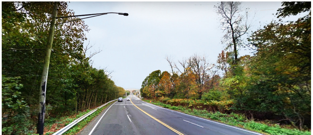
Route 59, westbound; Image credit: Google Street View
